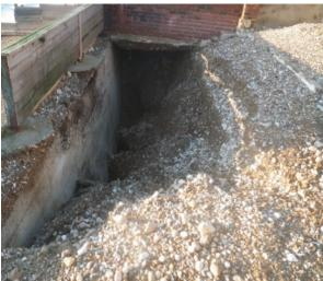
Emergency repair works were carried out to a 75m section of defences following two failures to the concrete apron, located on Selsey West Beach. Following failure of the seawall apron, washout of material caused significant voids behind the sea wall. Multiple properties were at risk from the failure, with some properties situated just 10-12m behind the wall.
